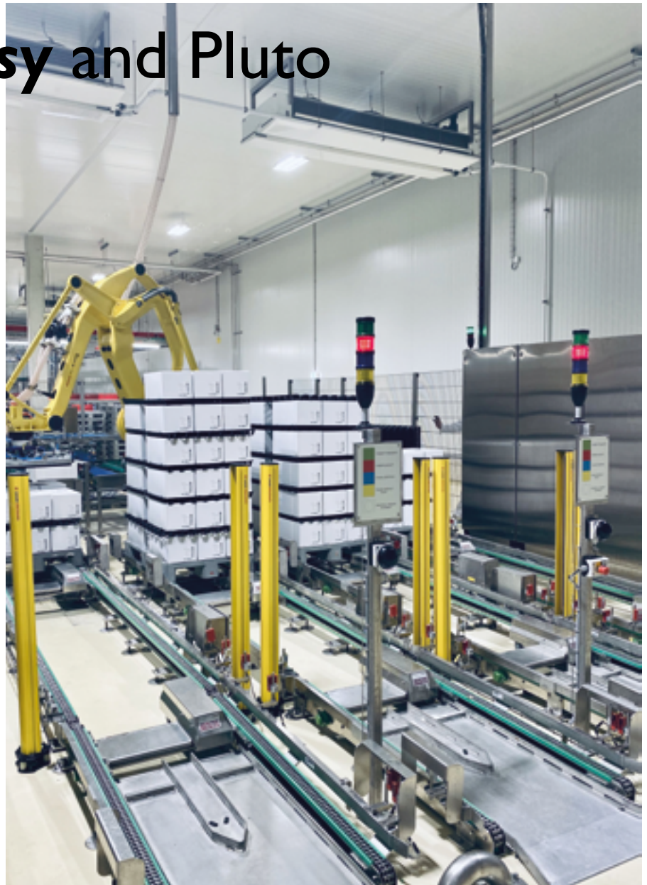
Quite futuristic: the new packing plant of Steirerfleisch in Styria.
